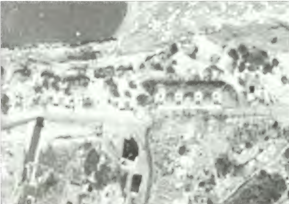
Figure 5.28. Aerial photograph of Batteries Urmston and Morris, January 1933. This photograph indicates that at this time, the concrete surfaces belonging to Batteries Urmston and Morris did not feature a paint, asphalt emulsion, or another darkly hued surface treatment (Coastal and Hydraulics Laboratory, Engineer Research and Development Center).
